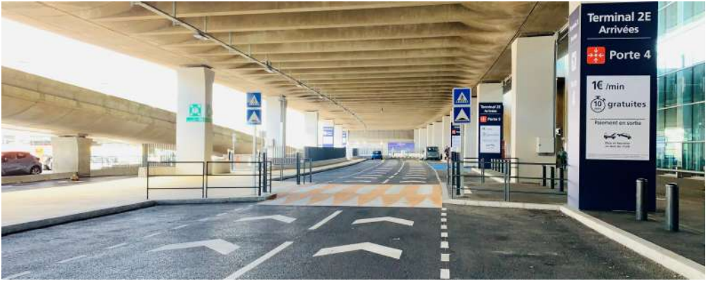
View of the Terminal 2E drop-off area at Paris-Charles de Gaulle, on Arrivals level, looking towards entrance 5. © Isabelle Vetter for Groupe ADP.
