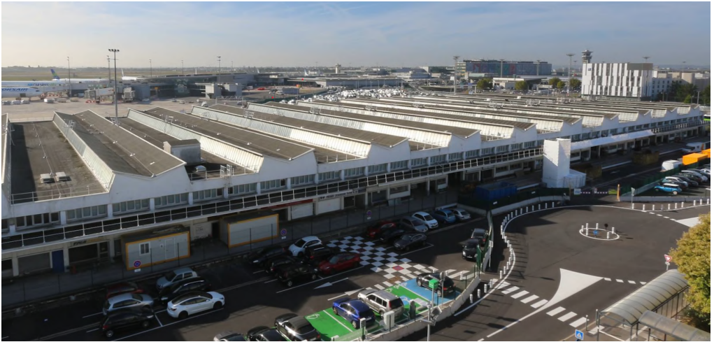
View of Building 351 before its demolition. © Premys for Groupe ADP.
