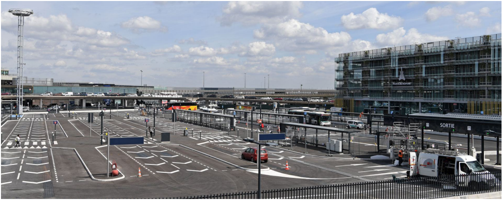
View of the revamped esplanade at Orly 1,2,3. © Sébastien Aubry for Groupe ADP.
